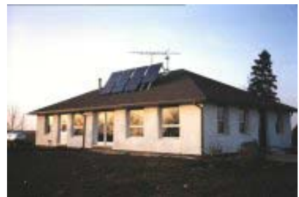
a Stelle straw bail solar powered home
